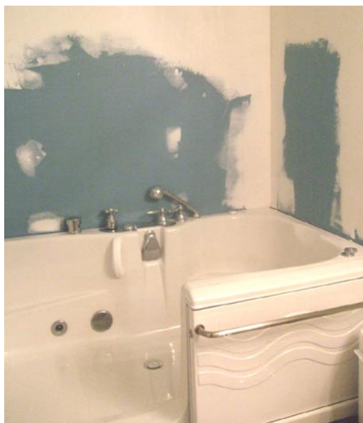
Installing aquaboard before final surround or tile.
