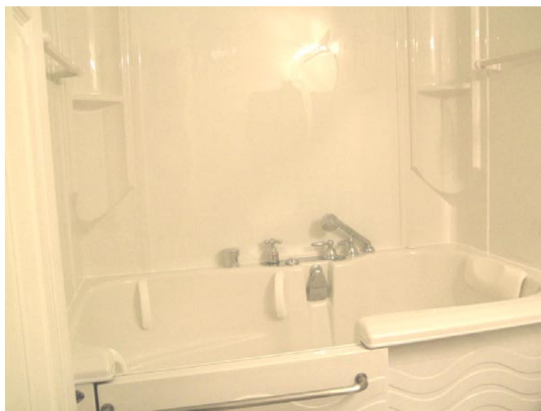
Installation complete with surround.
