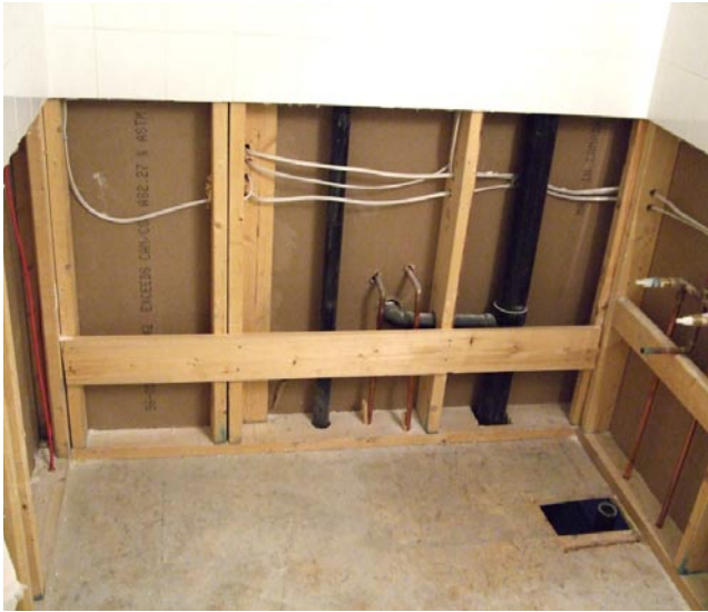
Original bathtub removed from alcove.
