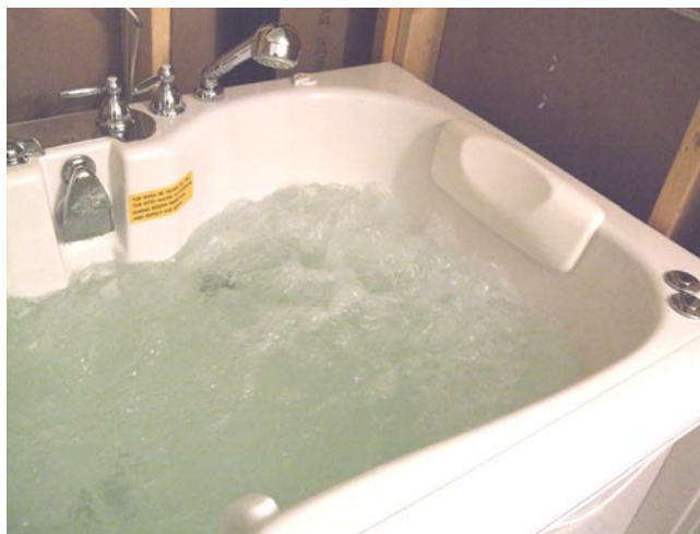
Final testing of air and water jet systems before enclosing tub installation.
