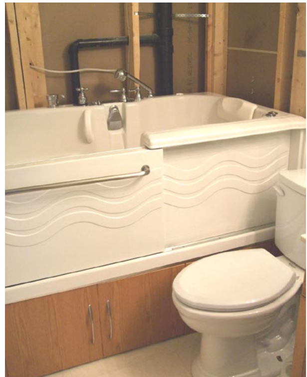
Toilet replaced. Bathtub operational.
