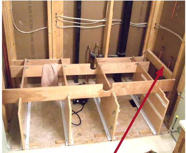
Frame for cabinet base being installed
