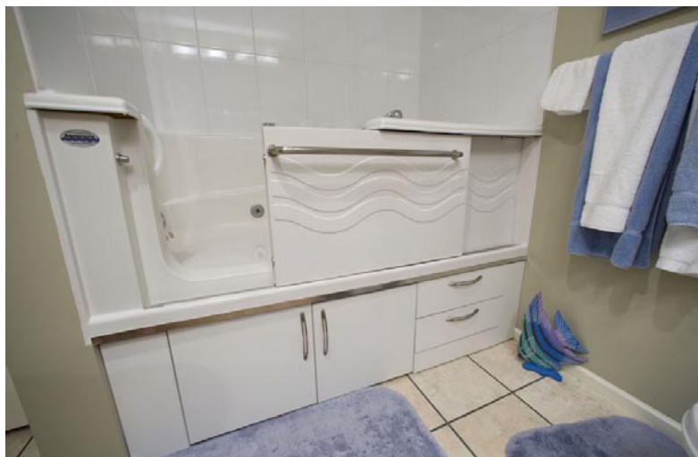
A finished installation with tile.
